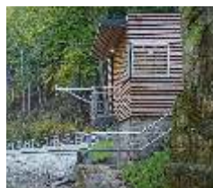
water level with radar sensor
