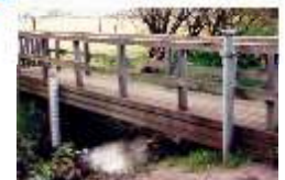
water level measurement with pressure sensor
