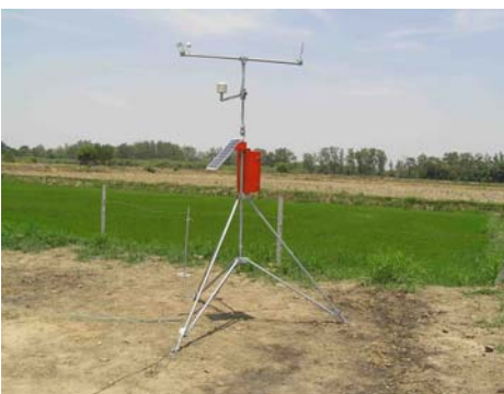
Weather Monitoring System installed at Kanpur (UP)
