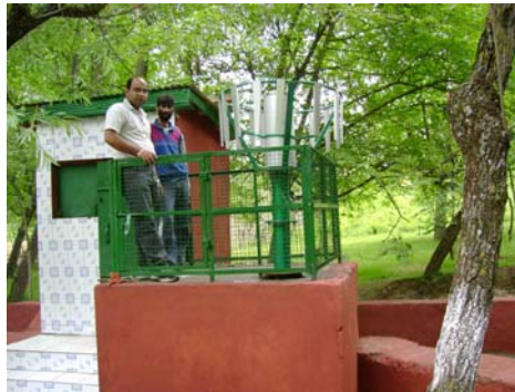
Hydrological observatory installed at Srinagar, J&K (India)
