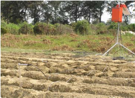
Automatic Soil Tensiometer installed at Varanasi (UP)
