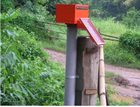
Automatic Water level Recorder installed at Bernihat Meghalaya, India
