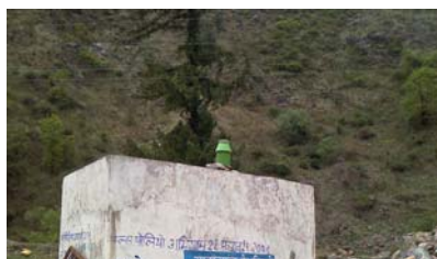
Digital Rainfall Recorder installed at Uttarakhand
